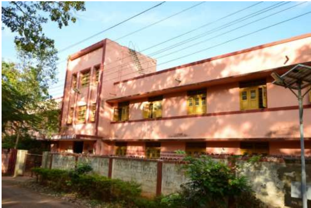
Picture 10. The Kaveri Hostel (Building 1) for residence of Girl students belonging to KSCD and KACD
